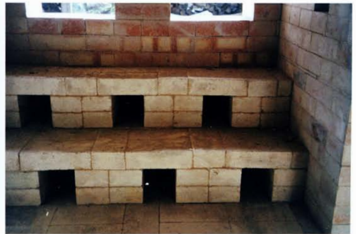
Interior of the anagama firebox, step-grate with air ports under each step. Photo credit: Tony Moore.
